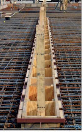
The entire surface of the slab was pitched to trench drains like the one shown here. As a result, much of the slab had to be "hand struck."
