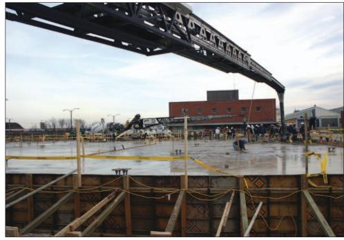
Above: This  $4^{1/2}$ -foot-thick mat slab will support a coal-fired generation plant with a boiler weighing more than 6 million pounds. Right: The precision location of anchor bolts was one of the most important elements of this project (see Fig. 1, p. 3). Lindblad placed "mud mats" to hardware for holding the anchor bolts in position during placement. Notice the steel mesh on top of the rebar, making it safer for workers to move around while concrete was being placed.
