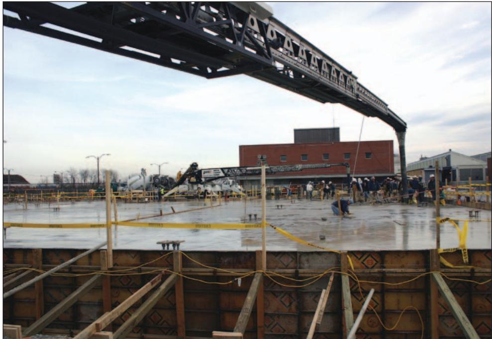
**Above:** This 4½-foot-thick mat slab will support a coal-fired generation plant with a boiler weighing more than 6 million pounds. **Right:** The precision location of anchor bolts was one of the most important elements of this project (see Fig. 1, p. 3). Lindblad placed “mud mats” to hardware for holding the anchor bolts in position during placement. Notice the steel mesh on top of the rebar, making it safer for workers to move around while concrete was being placed.
