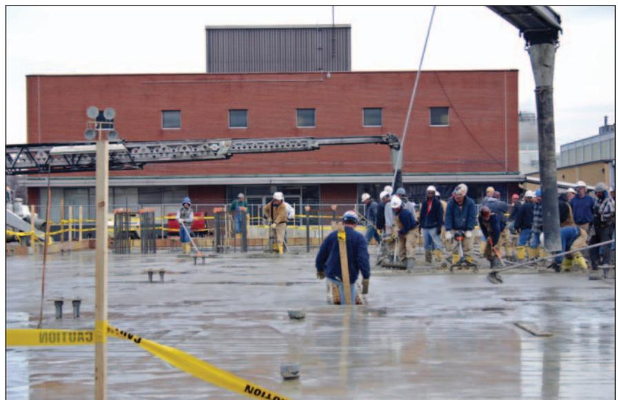
**Finishing concrete placement. Because the heat of hydration of the concrete mix was so low, finishers waited as long as 8 hours to begin finishing operations. Because of the pitches, the entire slab was finished by hand.**
