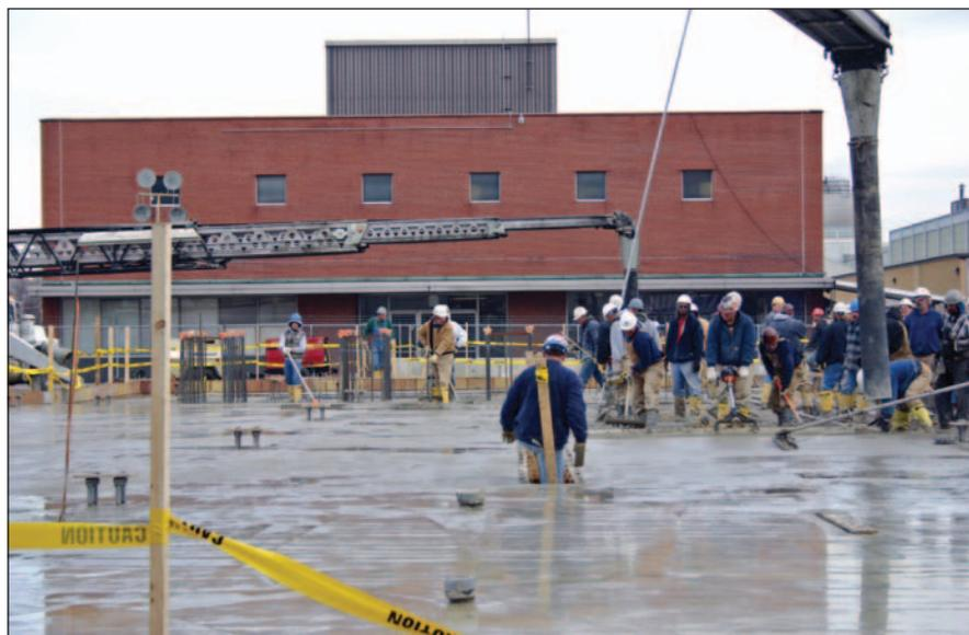
**Finishing concrete placement. Because the heat of hydration of the concrete mix was so low, finishers waited as long as 8 hours to begin finishing operations. Because of the pitches, the entire slab was finished by hand.**
