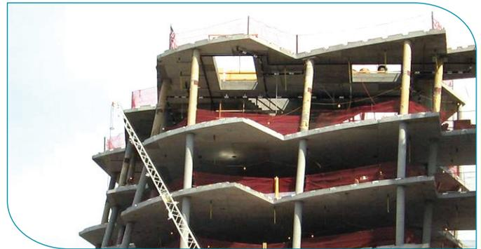
Fig. 1: Large opening in flat slab floor
