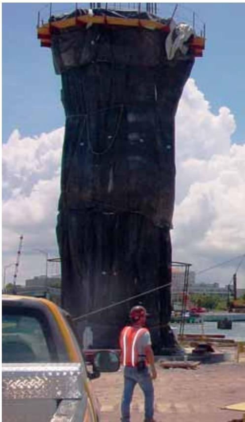
(left) A bridge column uses surface insulation to minimize the temperature difference between the interior and the surface.
